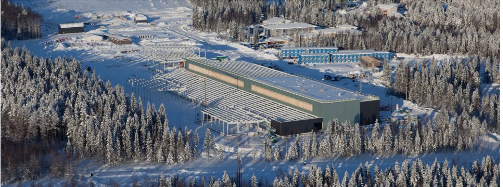
Facebook data center in Sweden.
