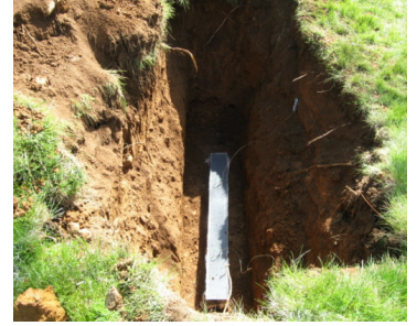
(c) Installed sensors in the box with temperature probes before burying
